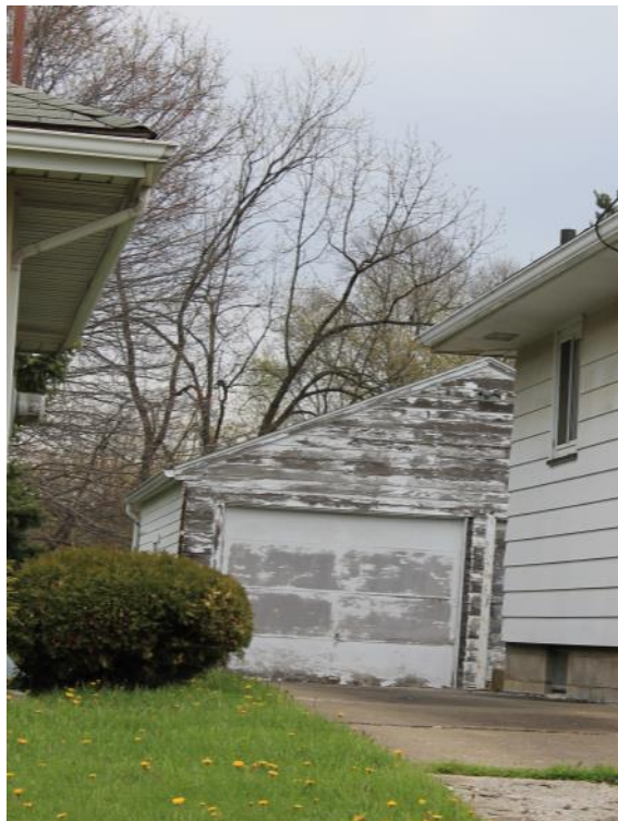
Peeling paint is a code violation
