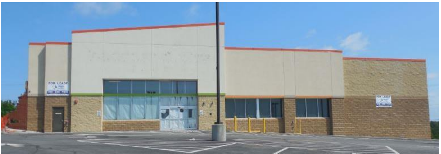
The former Bottom Dollar grocery store building is a key opportunity site for a new grocery store, as currently one does not exist on the Mahoning Ave. corridor.
