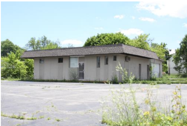
This building was likely previously used as a gas station or automobile repair shop and will require an environmental assessment
