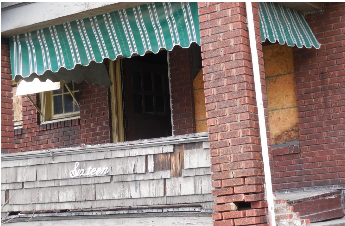
A blighted, vacant structure on Millet Ave. has a detrimental effect on surrounding properties
