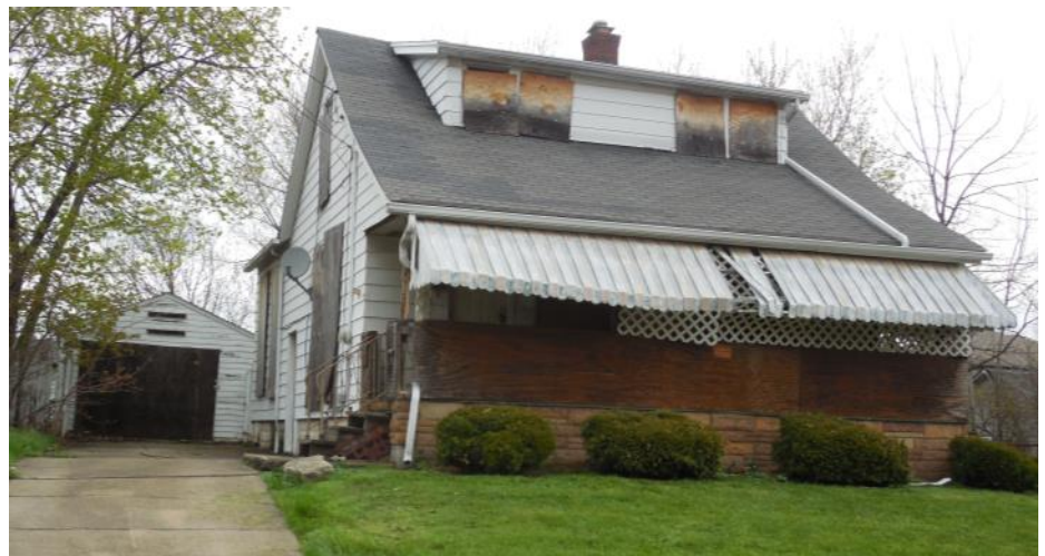
2218 OAKWOOD AVE: DEMOLITION
