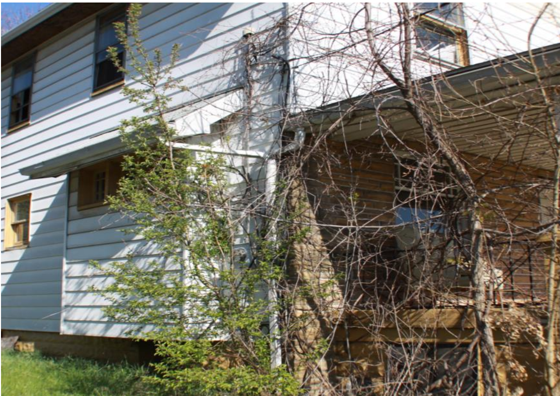
This vacant house on Millet Ave. should be cleaned up and the vegetation around the porch should be removed
