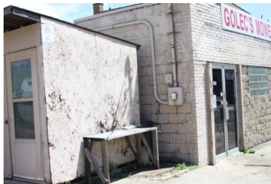
This building has peeling paint, which is a code violation
